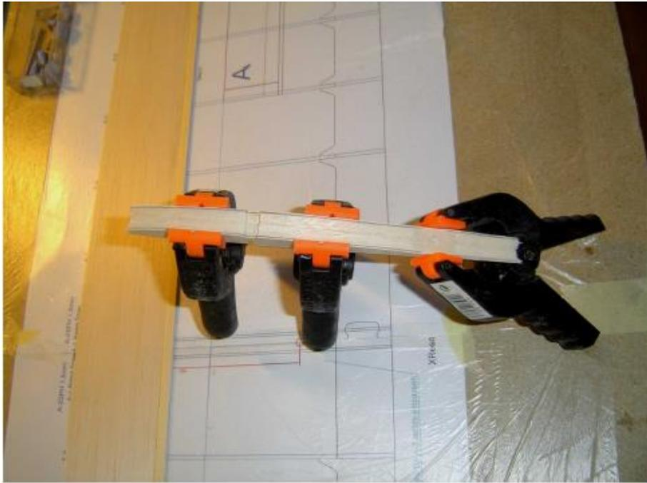
Ribs sorted on the plan and glued to spar. Do not glue ribs to bottom sheeting yet. Ribs A9 are glued at a 5 degree angle, using the 5 deg jig. See below. Make sure ribs are perpendicular. Use lots of glue around the spar and spar webbing.
